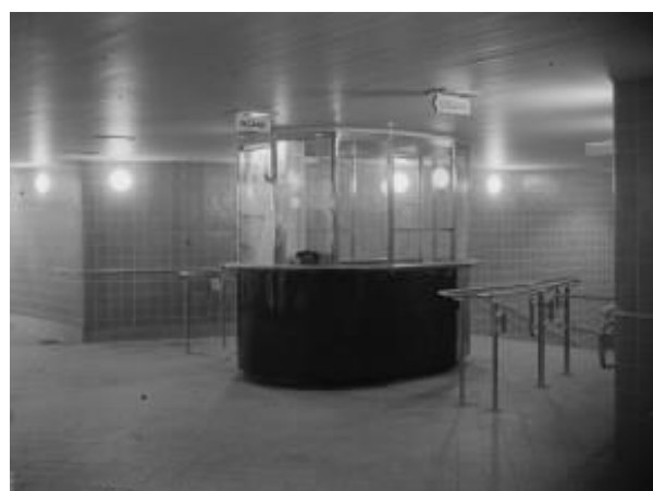
Figure 2. Södra Station Södra Bantorget, built according to the drawing. Source: Stockholmskällan. Photo: Unkown.
