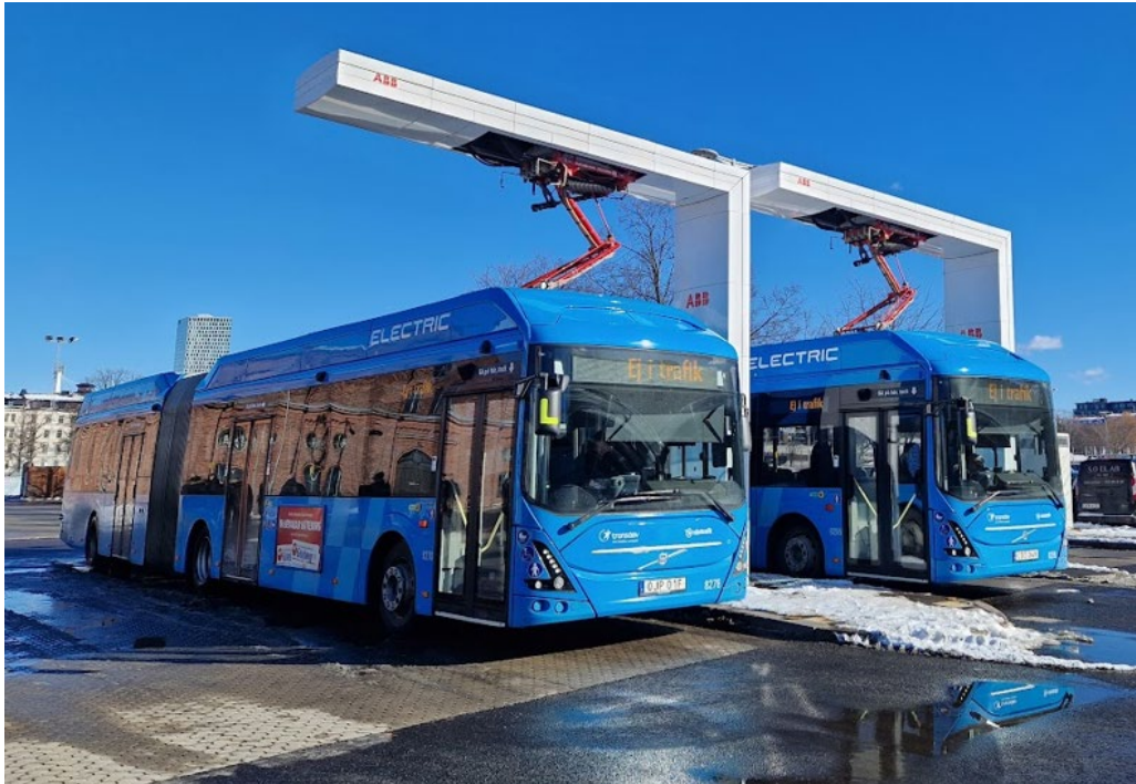
Figure 4. Buses charging using pantographs in Gothenburg
