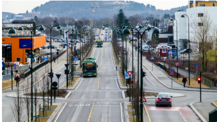
7:1) Physical separation of bus lanes using median refuges with trees in Stavanger, Norway. Image: PG Andersson, Trivector.
