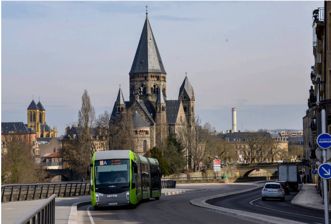
8) Bus lanes with both directions grouped together alongside the general traffic lanes in Metz, France. Image: PG Andersson, Trivector.
