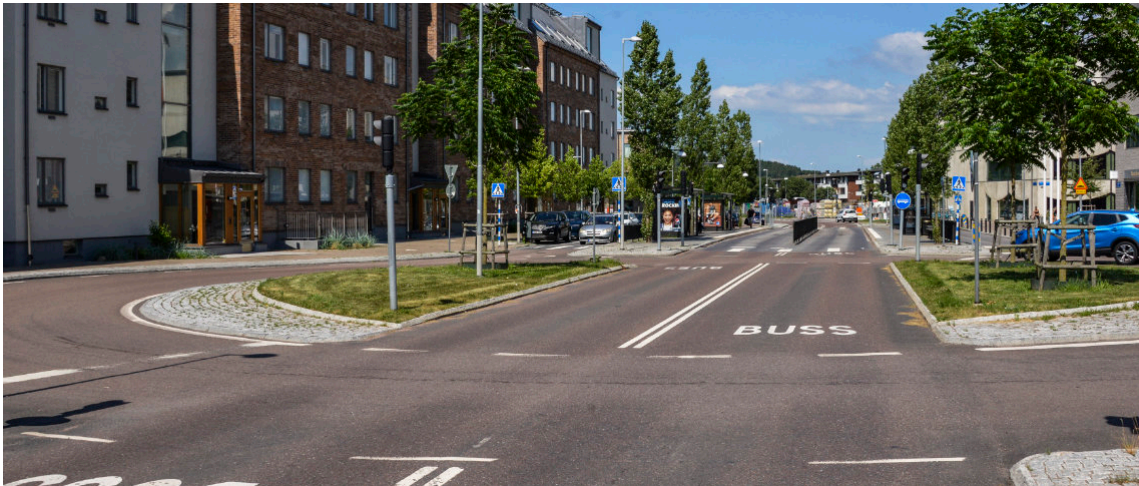
14:1) Litteraturgatan, Gothenburg. The bus lanes run straight through the signal-controlled roundabout, meaning that no crossing traffic occurs when the bus passes. Image: PG Andersson, Trivector.
