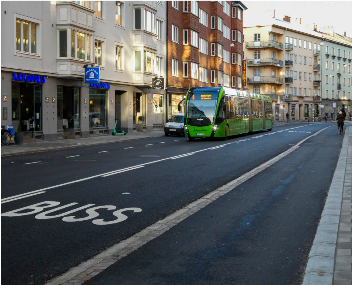
5) Davidshallsgatan, Malmö. Previously, buses shared traffic lanes with taxis and cyclists. As part of the reconstruction for MalmöExpressen, buses were given their own dedicated lane and cyclists a separate cycle lane, while taxi traffic was diverted to other streets. Image: PG Andersson, Trivector.
