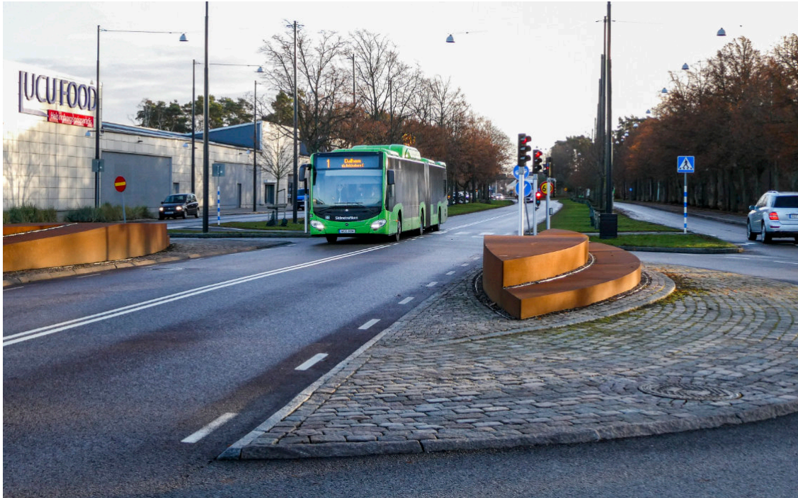
3) Straight through in Helsingborg: the busway runs directly through the roundabout, thereby avoiding three sharp curves – at the entry, within the roundabout, and at the exit. Image: PG Andersson, Trivector.
