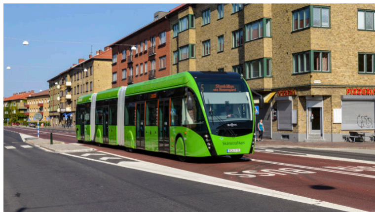
7:3) Visually marked bus lanes using red-coloured asphalt on Amiralsgatan in Malmö. Image: PG Andersson, Trivector.
