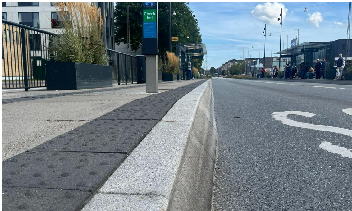
Figure 15. Along Line 2 in Aalborg, the stations feature 24-centimetre-high platforms to achieve platform-level boarding without bus kneeling. Platform extensions are also used. As a result, the busway is slightly narrower at station locations than along the sections in between.
